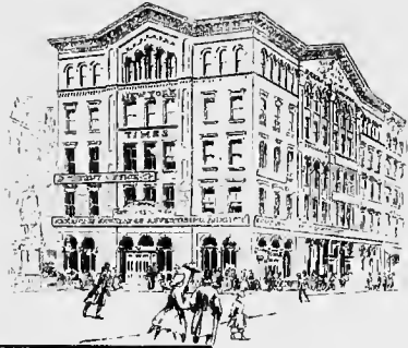
THE THIRD TIMES BUILDING. PARK ROW. 1857-1888.
